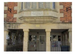
The stone is unfortunately a soft Cotswold limestone. It has been damaged by water running down the bay window above which is then channelled into the pillars. Recent cold winters have frozen water contained in the stone, which has then expanded, thus breaking the stone. The stone is literally crumbling. In some places water has penetrated and expanded cracks in the stone.
